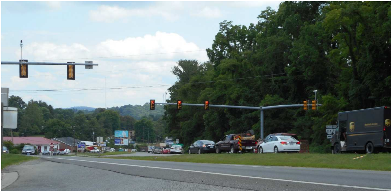
Lee Highway at Peppers Ferry Road intersection, looking north toward the City of Radford
