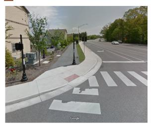
Features: Adjacent to traffic, generally shorter routes, convenient to more destinations along the corridor, grades generally consistent and match roadway slopes, generally less expensive and less ROW acquisition required to develop, generally takes less time to plan and construct.
