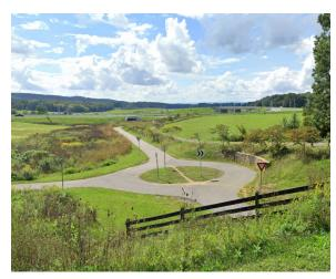
Features: Away from traffic, better for less confident cyclists, generally longer routes, destinations limited, grades change with the terrain and are generally more variable, generally more costly and can require extensive right-of-way acquisition, longer planning and construction timeline.
