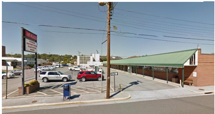
Figure 7: PAT Administrative Offices (top) and Town of Pulaski Shop (bottom)
