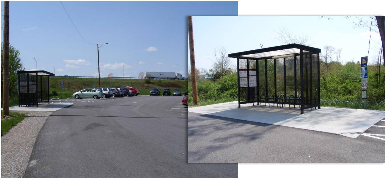
Park and Ride Stop (above); stop shelter/information (top right).
